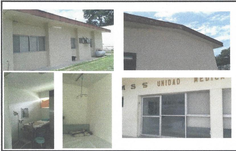
**DESCRIPCION:SE OBSERVAN FISURAS QUE NO AFECTAN A LA ESTRUCTURA , SE DETECTARON AFLOJAMIENTO DE AZULEJOS Y PISOS**
