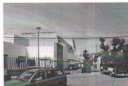
VISTA GENERAL DEL HOSPITAL
