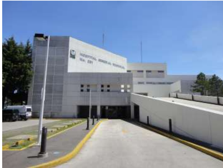
Foto 2. Vista de Fachada Lateral del Hospital General Regional IMSS-HGR No. 251
