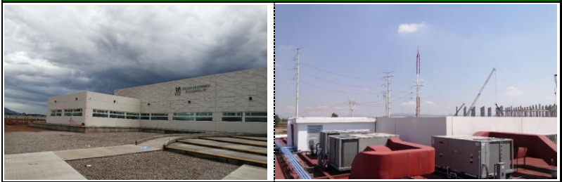
FACHADA PRINCIPAL UMF NO. 37
