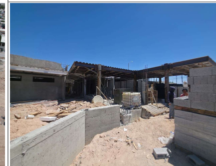
COLADO RODAPIE BARDA FRONTAL
