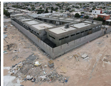
COLOCACION BLOCK BARDA PERIMETRAL
