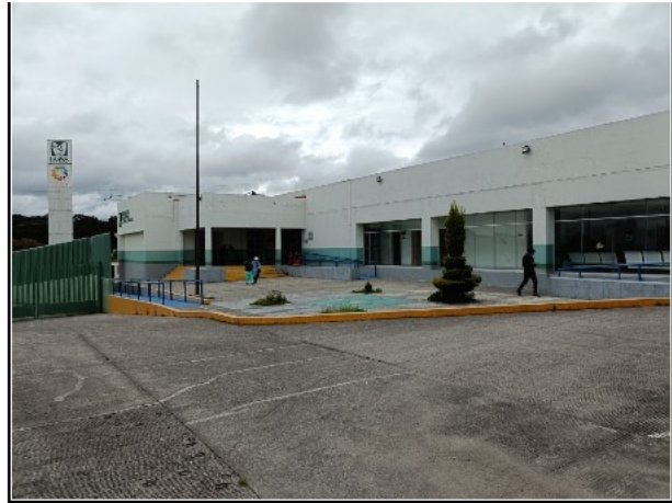
FACHADA INTERIOR DEL HOSPITAL
