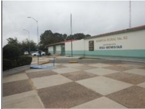
FACHADA FRONTAL HOSPITAL
