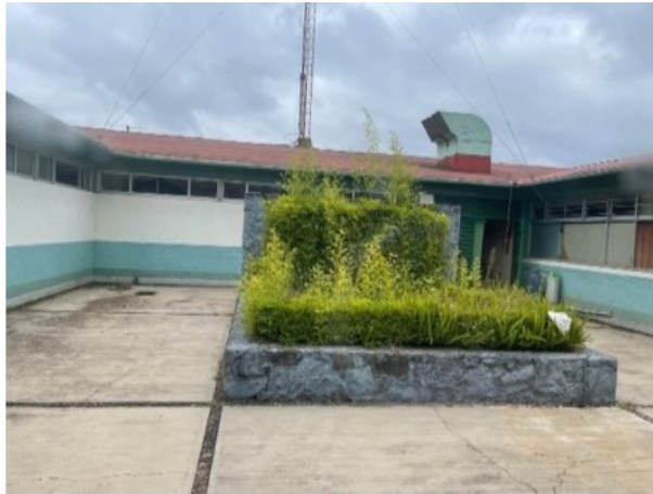
VISTA PATIO INTERIOR
