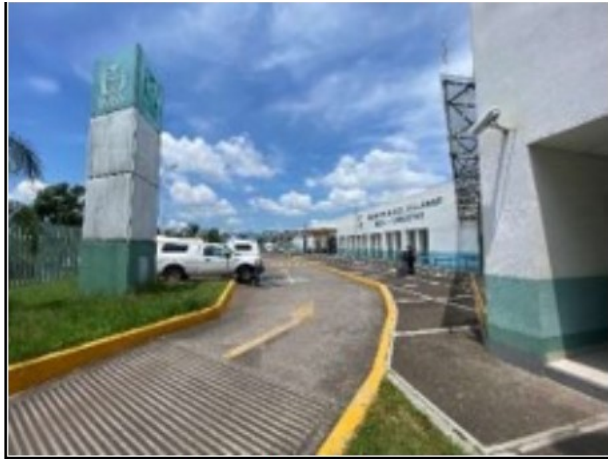
Exterior Hospital - Ingreso
