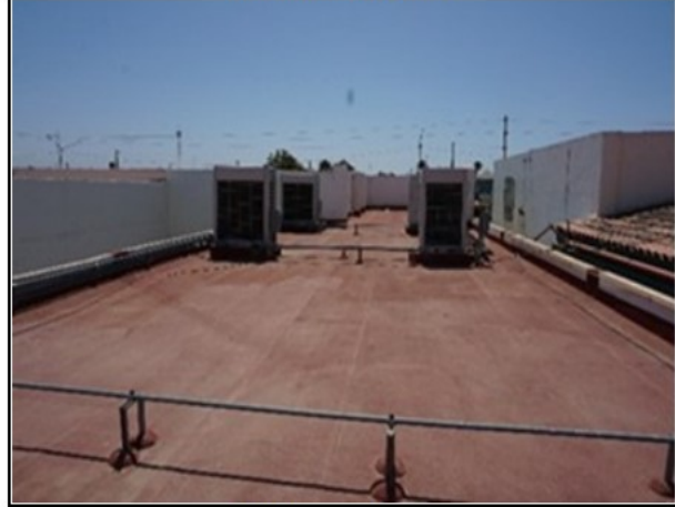
Vista general azotea
