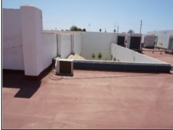
Vista general azotea
